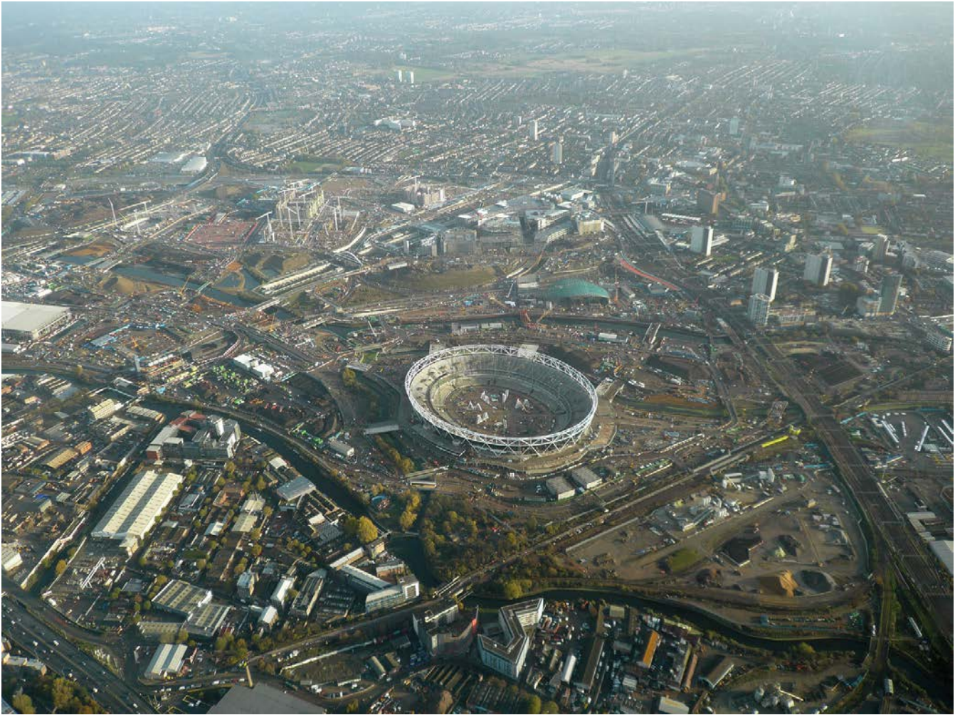
figure 9: London Olympic site in construction (Hackney Wick across the canal, bottom left), photo by Frans Zwart
